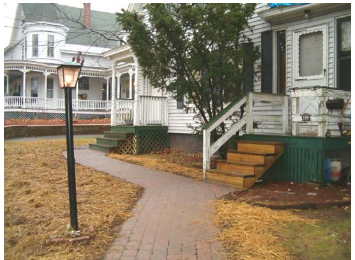
The New Walkway at 199 Washington Street
