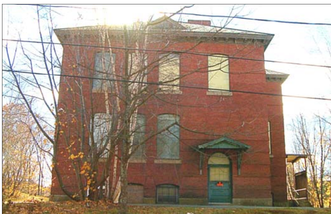
Mechanic Street School Building
