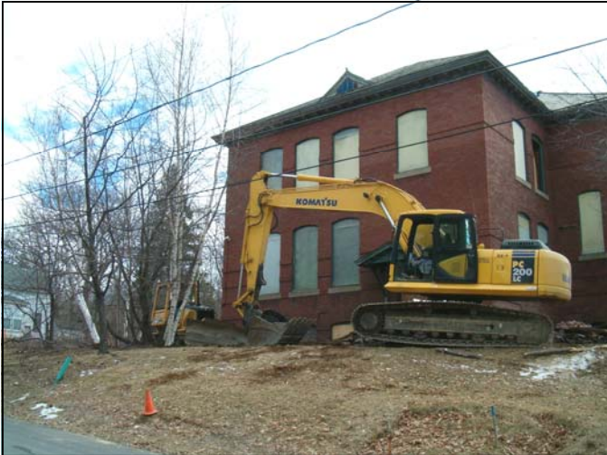
Site work underway at the former Mechanic Street School.
